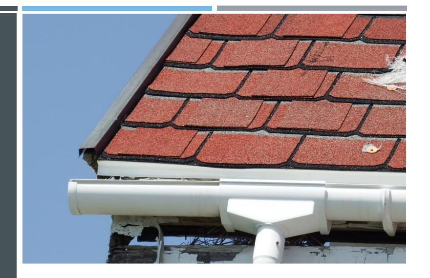
Water, moisture, and wind damage have accelerated paint peel
