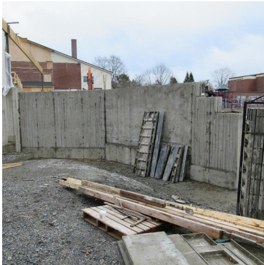
Playground Retaining Wall
