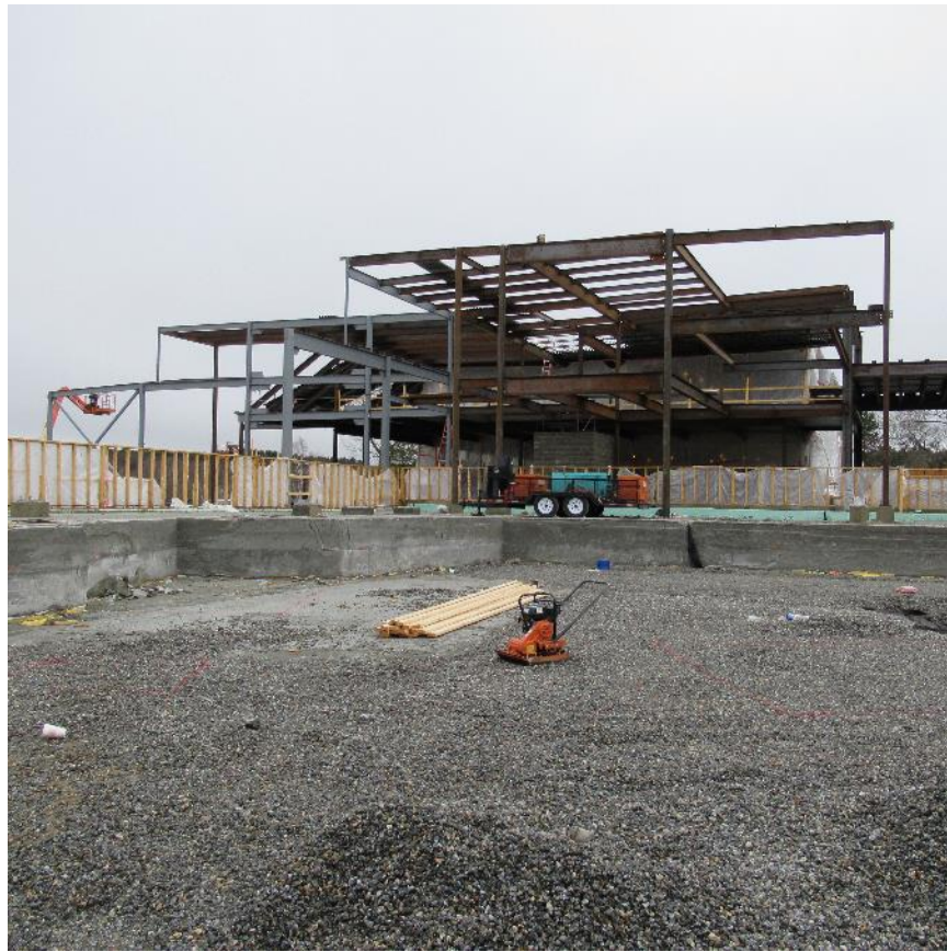
Looking West from Lobby
