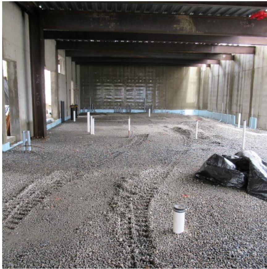
Mechanical Room Prepped for Slab
