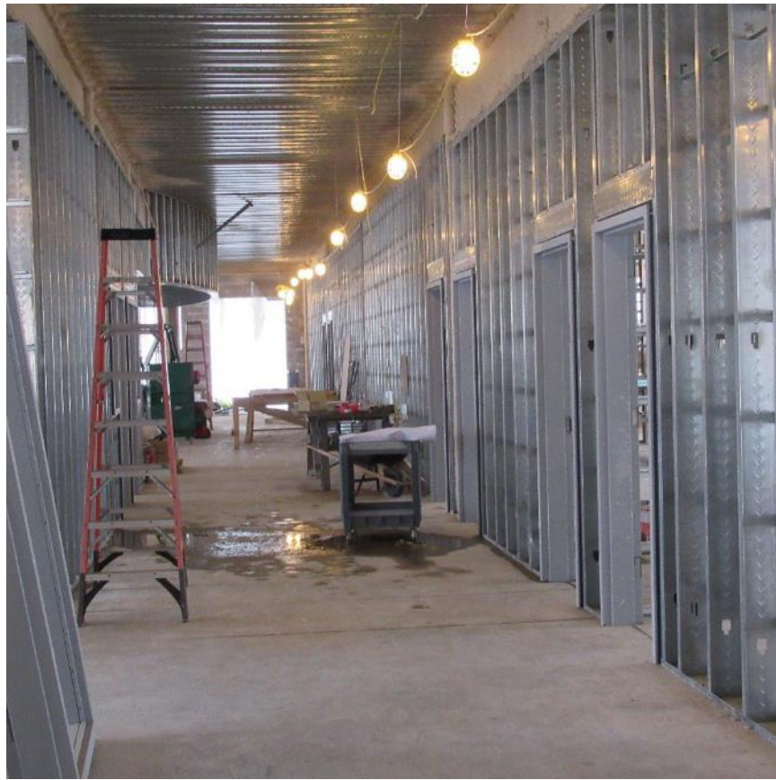
Lower Level Wall Framing at Classrooms
