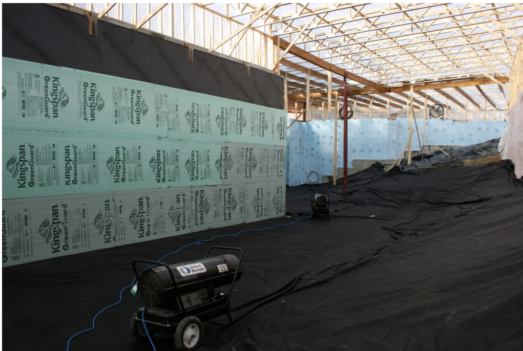
View behind the retaining wall, ready for cellular fill.
