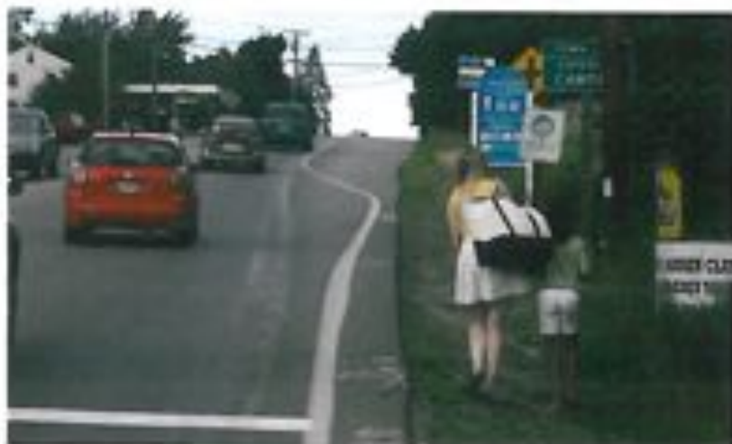
Fig. 3: On Elm Street (Route 1) near Camden town line, at the signal, looking north. Arriving bus passengers are walking into town. Note lack of shoulder after recent MDOT redesign of traffic flow. The proposed project plans to widen this breakdown area.
