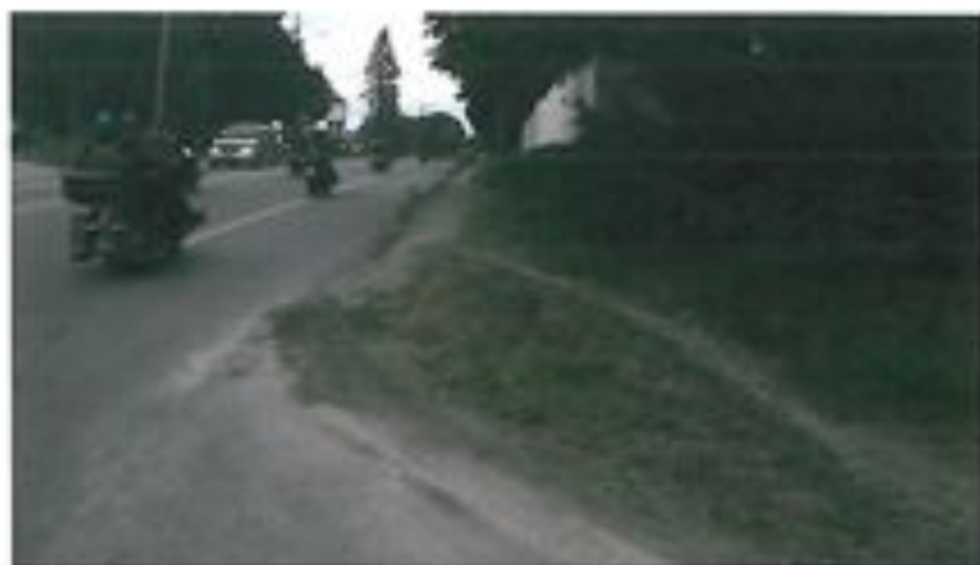
Fig. 10: Northern end: the present terminus of the sidewalk, seen here on the northeast corner of Camden St. (abutting Quarry Hill adult community) is narrow, not easily negotiable, unpaved and drops 15" to the road. Proposed sidewalk will remedy this and complete much-needed pedestrian connections to Quarry Hill adult community (82 cottages & apts, 60 asst'd living residences, 135 staff) and to multiple Inn's and downtown Camden.
